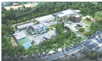
Gongsan Drinking Water Treatment Plant in Daegu Client ----- Daegu City Capacity ----- 40,000m 3 /day
