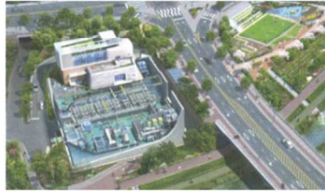
Siheung Mokgam Sewage Treatment Plant Client ----- Siheung City Capacity ----- 13,000m 3 /day
