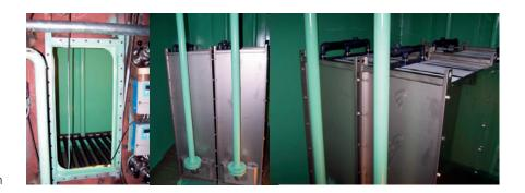
Pictures showing Sewage treatment system with aeration tank and Membrane-bio-reactor tank with the MicroClear® Filter housing installation
