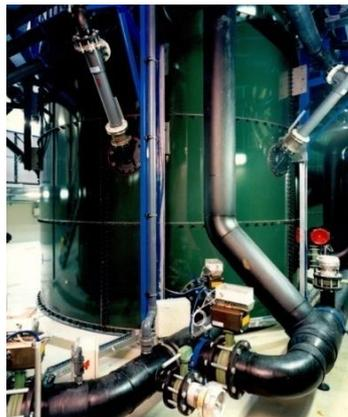
In order to avoid that valuable biomass is washed out along with the water, the microorganisms are entirely held back by means of a cross-flow microfiltration technique and are then recirculated to the unit.
