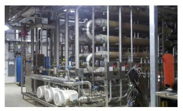
Picture 1. External AnMBR system with Berghof Membranes UF modules
