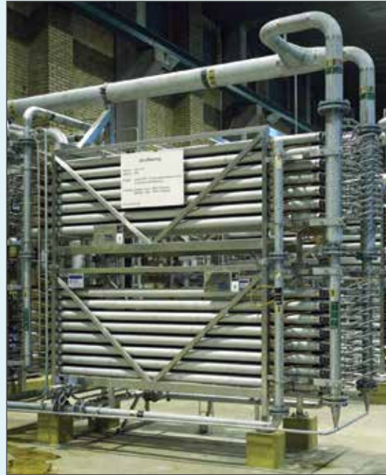
View of feed end of sixth stage of hardwood line. Note: Larger diameter feed pipework
