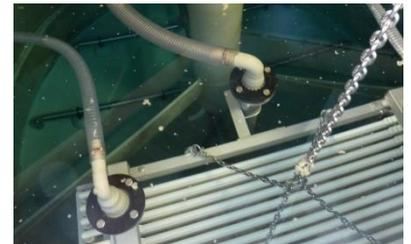
Possible changes in sludge quality as well as high hydraulic loads do not cause a loss of biomass due to wash out. The reduced space requirements in comparison to conventional activated sludge processes with a final sedimentation basin is an additional advantage especially for existing industrial plants with limited space.
