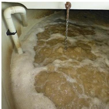
The biological treatment takes place in the MBR tank. Due to the membrane, all biomass in the form of activated sludge is held back and therefore, the sludge age can be freely chosen. Aeration on the bottom of the tank ensures aerobic degradation of organic substances, as well as prevents sludge particles from clogging the membrane. Heavy metals and persistent organic substances are eliminated by accumulation in the activated sludge.
