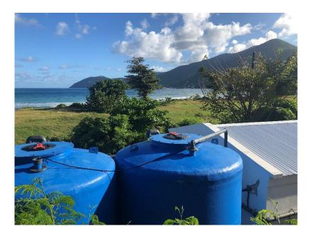
Respecting the coastal location of the resort, only non-metallic and corrosion resistant (316SS) materials were used to ensure the longevity of the system.
