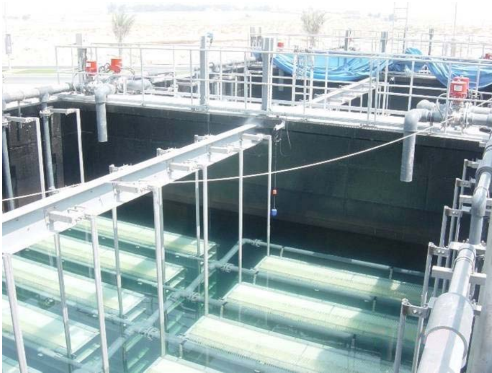
Typical view of the installation of MBR units
